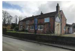
Fig. 10: North Elevation on to Kirby Misperton Road
